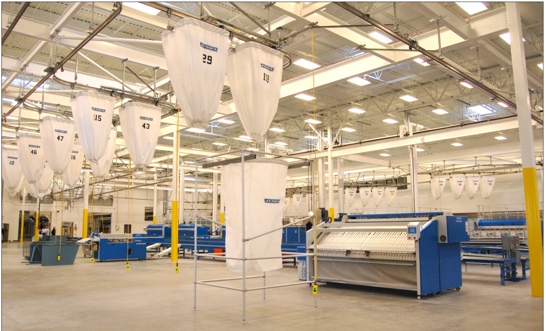
Equipment and staff in the new 146,000-square-foot laundry will wash, dry, sort and fold materials.
